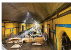
East Side Access Project, New York
